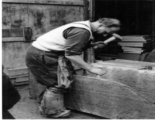
Fig. (6.4). Coarse-grained “greenslate” being split by hand for facing stone, England.
