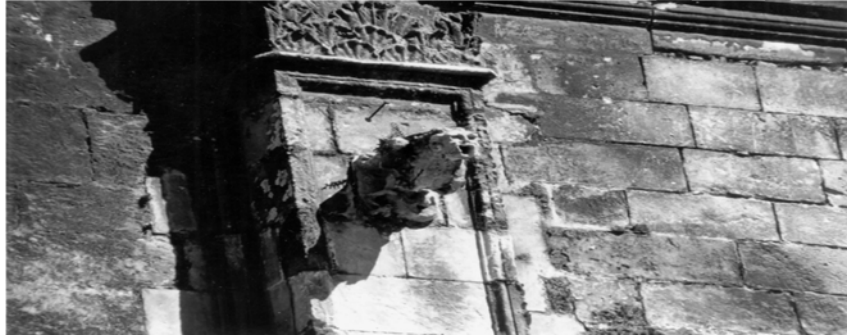
Fig. (6.3). Weathered limestone gargoyle and scabbing of stone, Seville cathedral, Spain.
